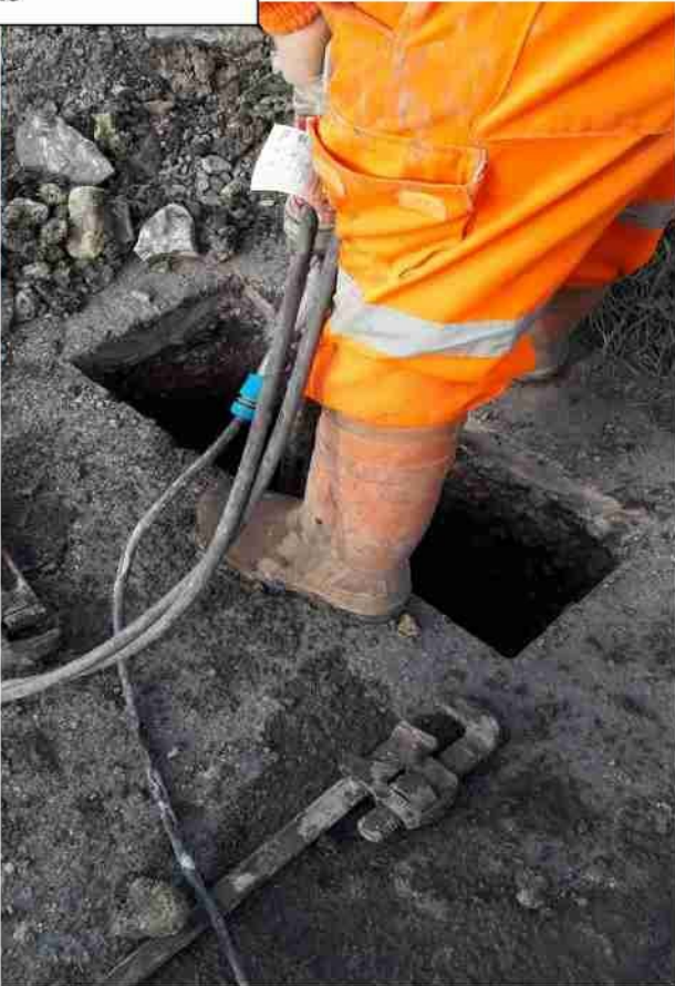
Extending coring bit to reach into concrete
