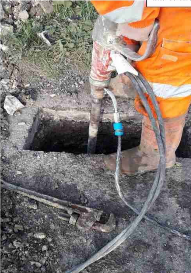
Extending coring bit to reach into concrete
