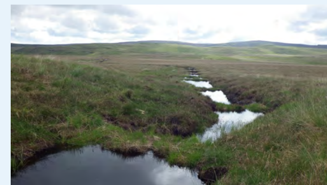
Figure 17 – A series of constructed peat dams in a moorland setting (© Moors for the Future Partnership)
