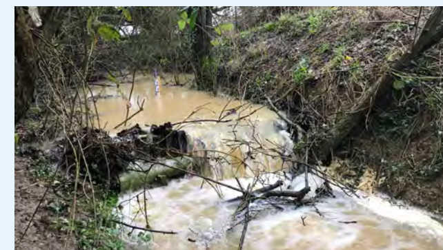
Figure 15 – Fixed large wood in-channel leaky barrier storing water during high flow event (© Dave Gasca-Tucker)
