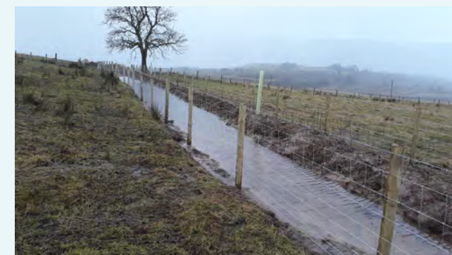
Figure 14 – A cross-slope swale with low-level bund on the downstream slope (© West Cumbria Rivers Trust)
