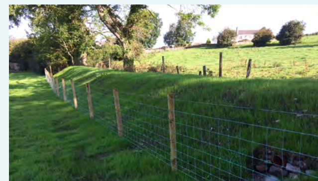
Figure 11 – A cross-slope bund with fence for added protection against livestock poaching (© Cumbria County Council)
