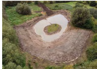
Figure 1. A newly constructed offline storage pond as part of the River Soar NFM pilot scheme (© Atkins Ltd)
