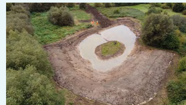
Figure 12 – A newly constructed offline storage pond as part of the River Soar NFM pilot scheme (© Atkins Ltd)
