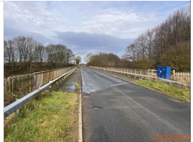
03. View west over deck.JPG
