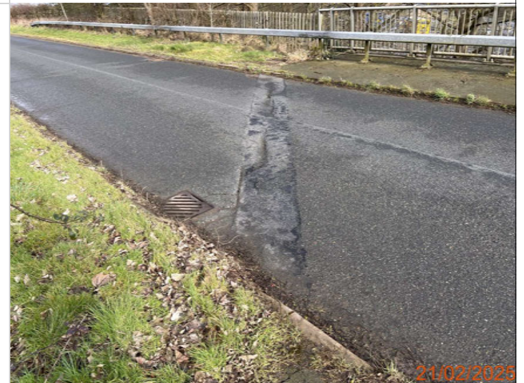
19. West abutment joint.JPG
