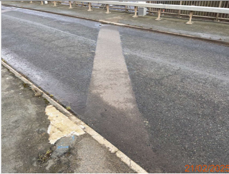
22. Southbound hinge joint - west.JPG
