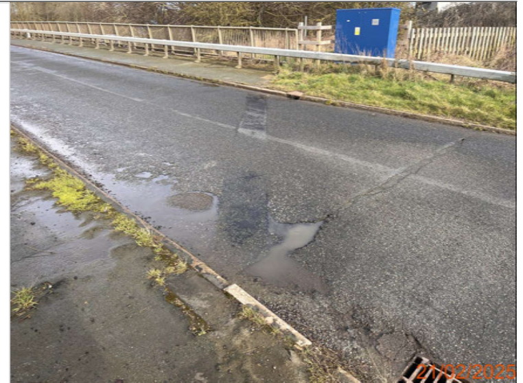
24. East abutment joint.JPG
