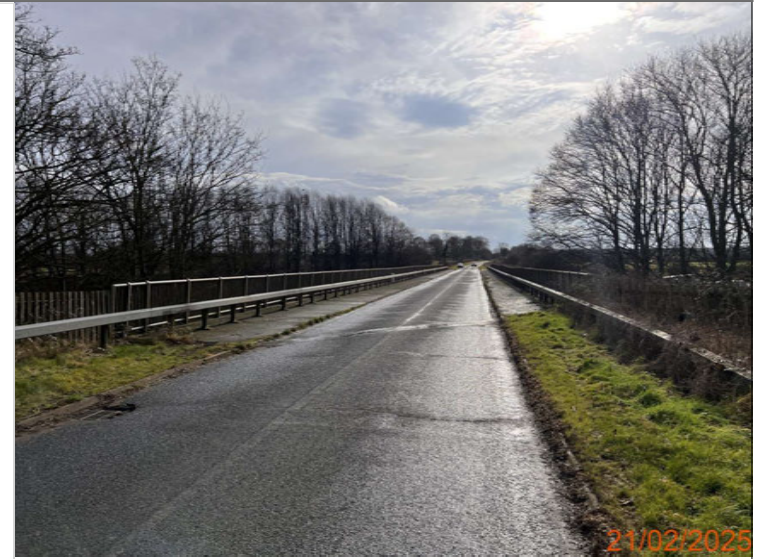
04. View east over deck.JPG
