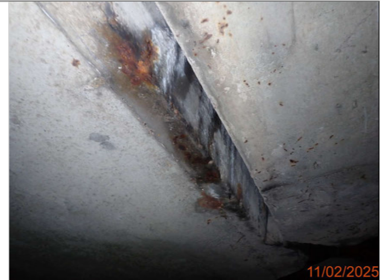
Water and leachate staining to the west hinge joint over NB L1.JPG
