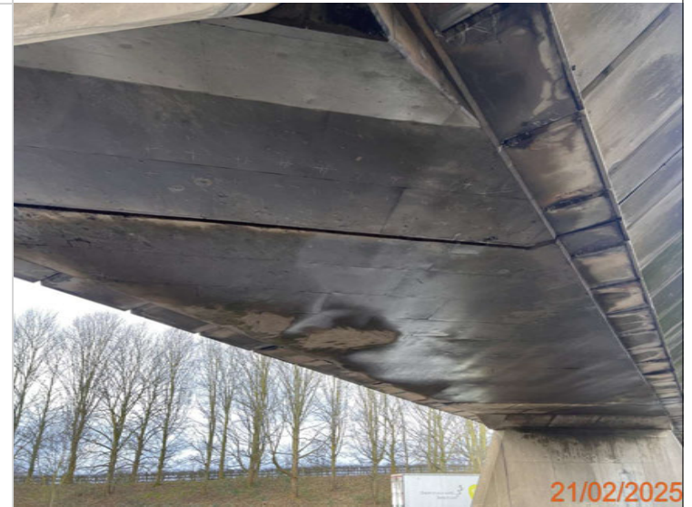
17. Southbound - east span soffit.JPG
