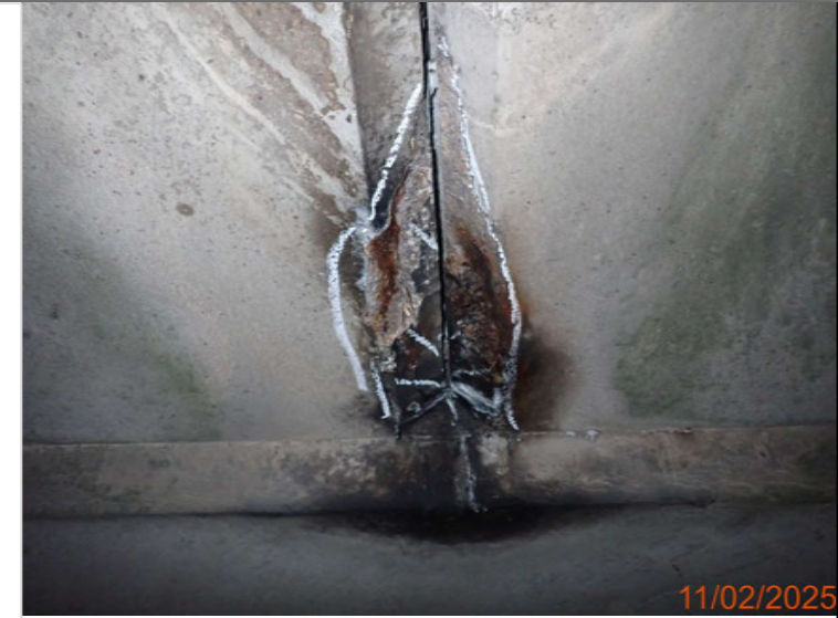
Spalling to the south service bay over NB L1-2 - 510 x 90 x 50mm.JPG
