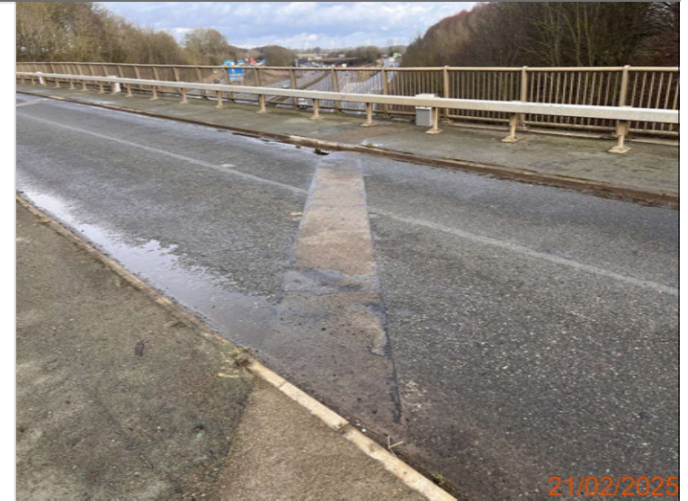
23. Southbound hinge joint - east.JPG
