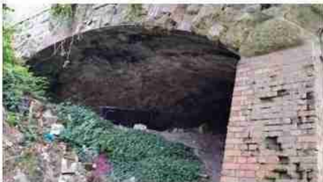
Plate 1 Arch 1 infilled on northern eastern facing side only
