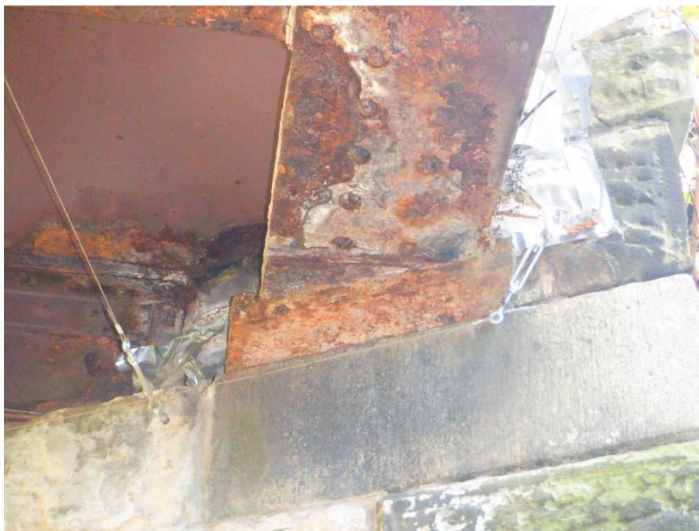
Photo No.8. East elevation parapet girder corrosion
