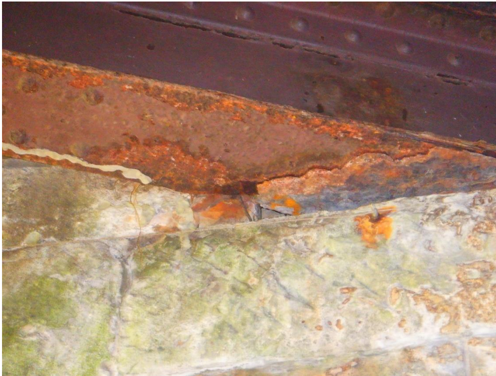
Photo No.13. Cross girders corrosion
