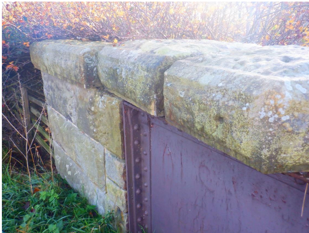
Photo No.17. South West elevation pilaster displaced
