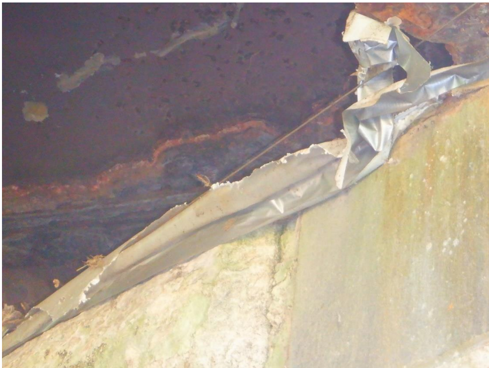
Photo No.14. Cross girders corrosion web plate holed at abutment not visible covered with polythene
