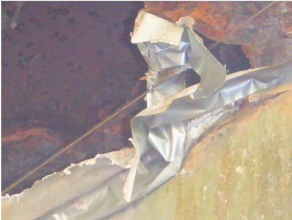
Photo No.15. Deck plate holed covered with polythene
