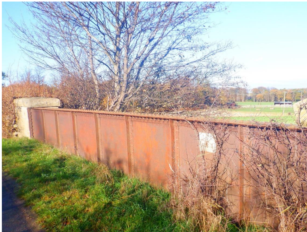
Photo No.7. East elevation parapet girder road face
