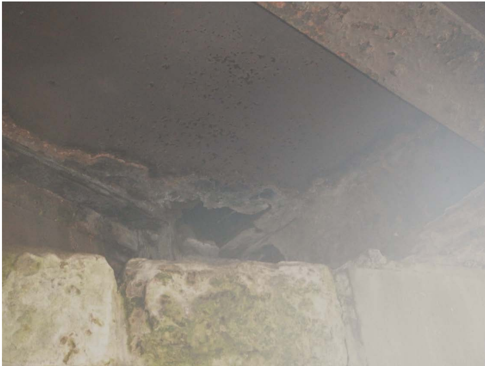
Photo No.15. Deck plate holed
