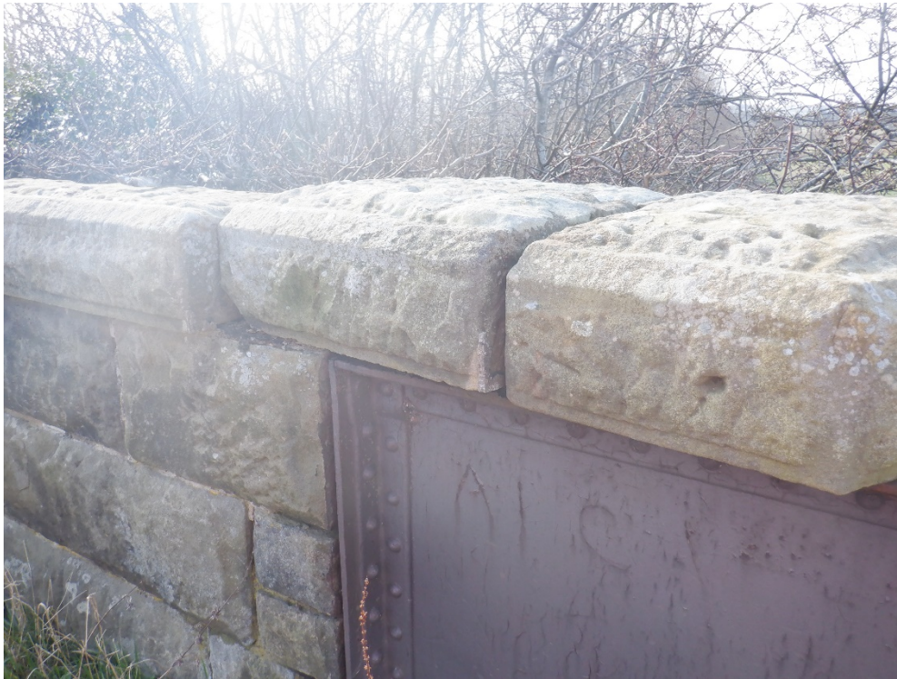
Photo No.17. South West elevation pilaster displaced
