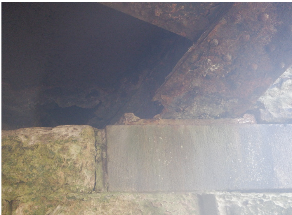
Photo No.12. West elevation parapet girder bottom flange notched
