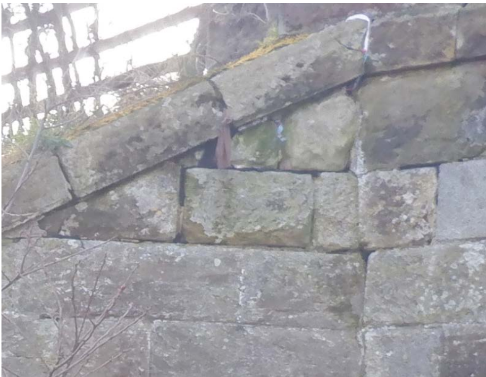
Photo No.16. South East elevation wing wall open joints
