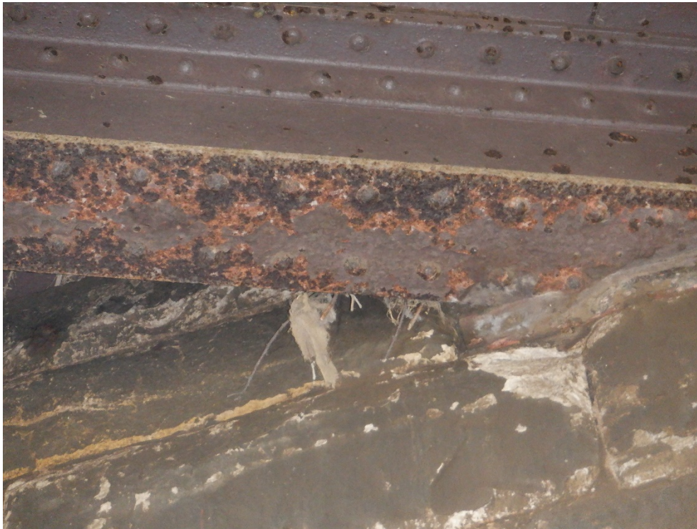
Photo No.13. Cross girders corrosion
