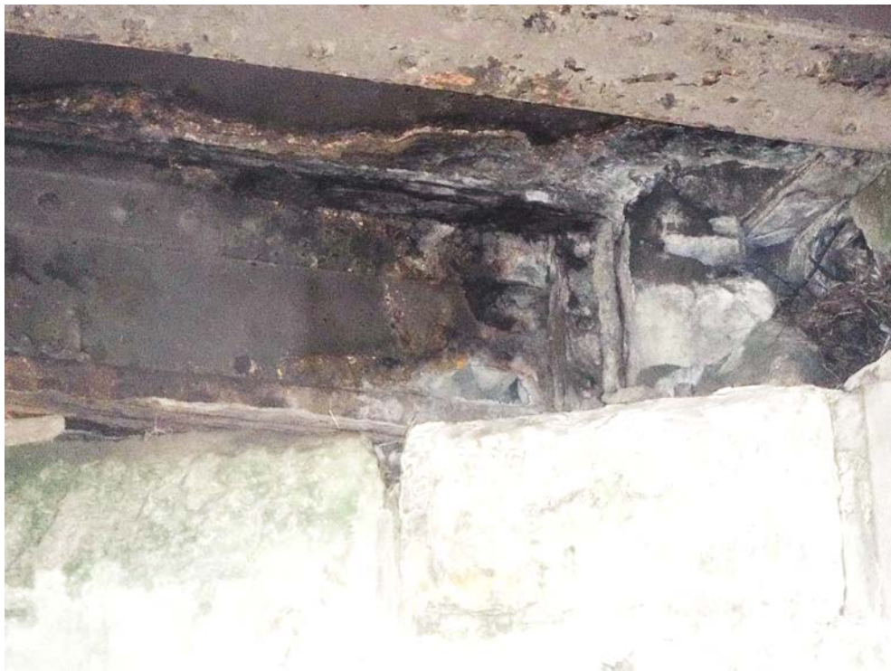
Photo No.14. Cross girders corrosion web plate holed at abutment
