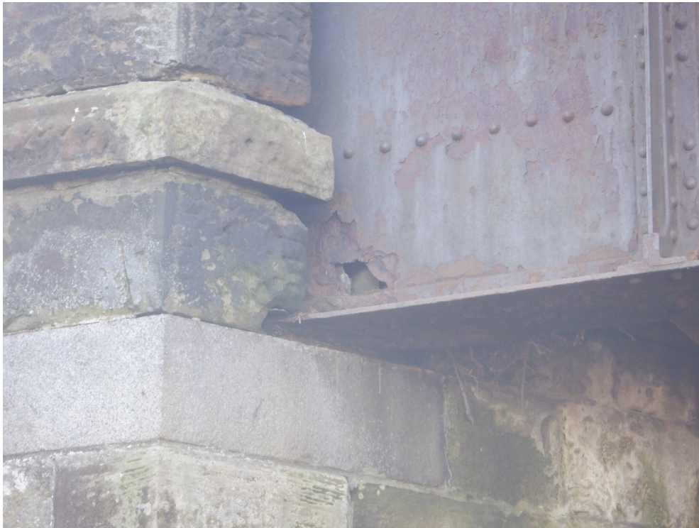
Photo No.9. East elevation parapet girder web plate holed
