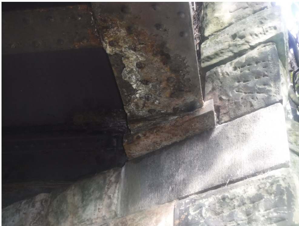
Photo No.8. East elevation parapet girder corrosion
