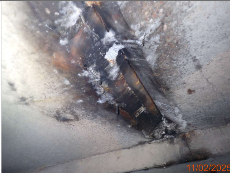
Leachate emanating between the north service bays over SB L1.JPG
