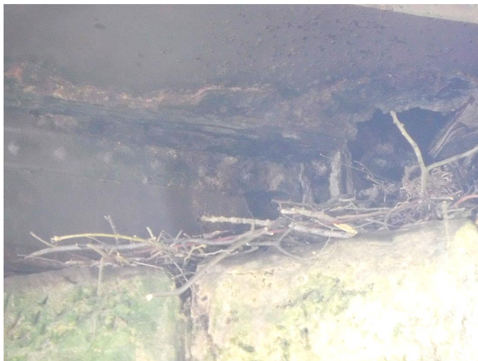
Photo No.11. Cross girders corrosion at abutments
