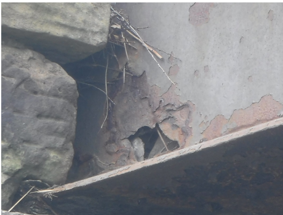
Photo No.7. East elevation parapet girder corrosion
