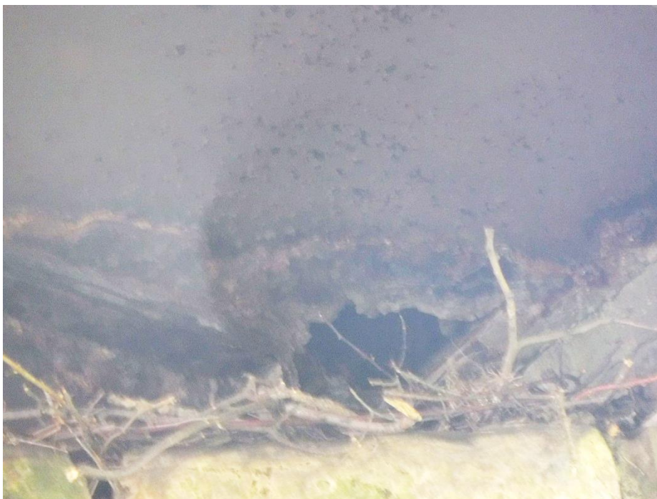
Photo No.13. Deck plate holed
