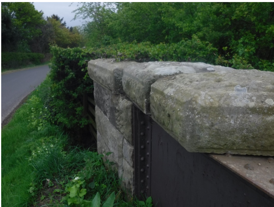
Photo No.15. South West elevation pilaster displaced
