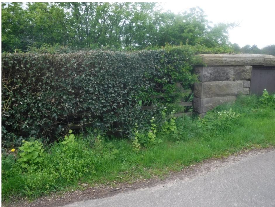
Photo No.15. South West elevation pilaster displaced
