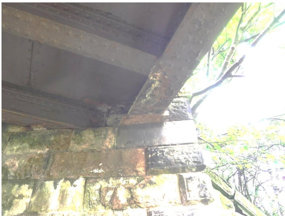
Photo No.7. East elevation parapet girder corrosion
