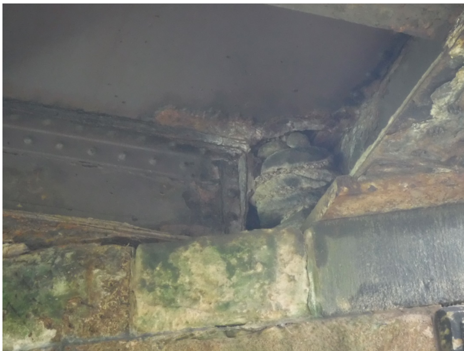
Photo No.11. Cross girders corrosion at abutments
