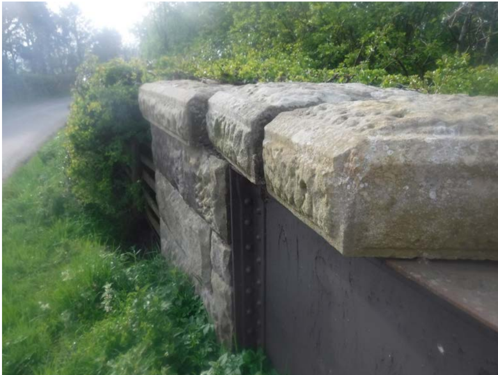
Photo No.17. South West elevation pilaster displaced
