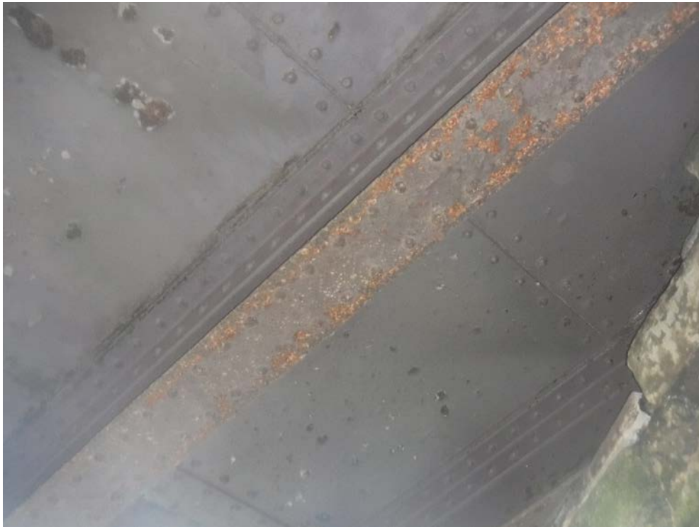
Photo No.13. Cross girders corrosion
