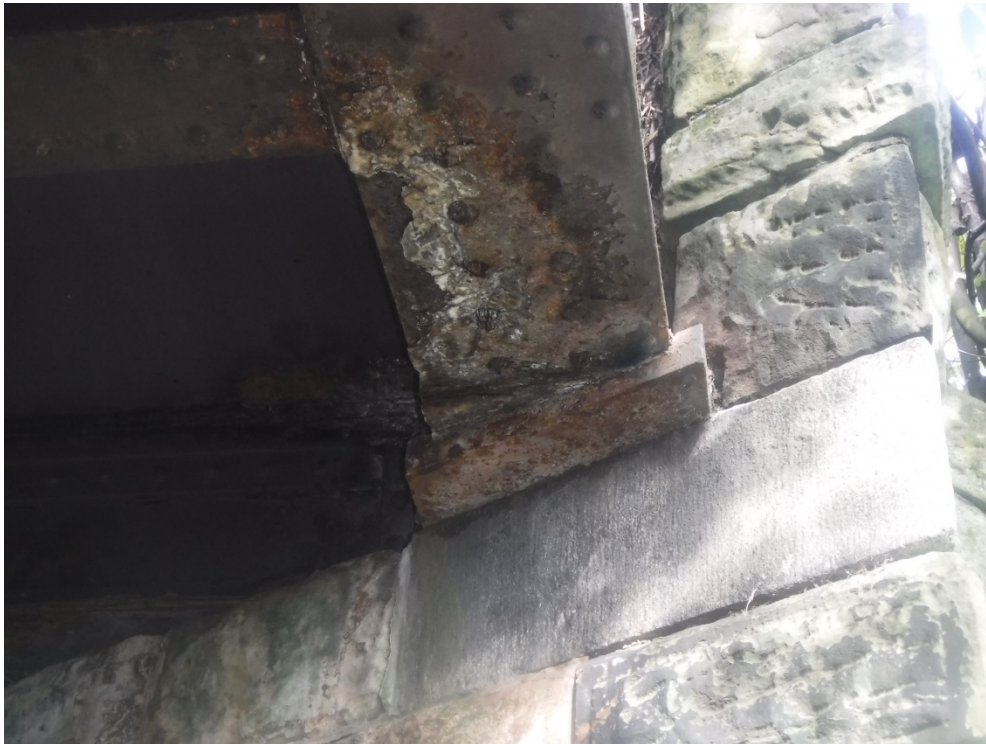
Photo No.8. East elevation parapet girder corrosion
