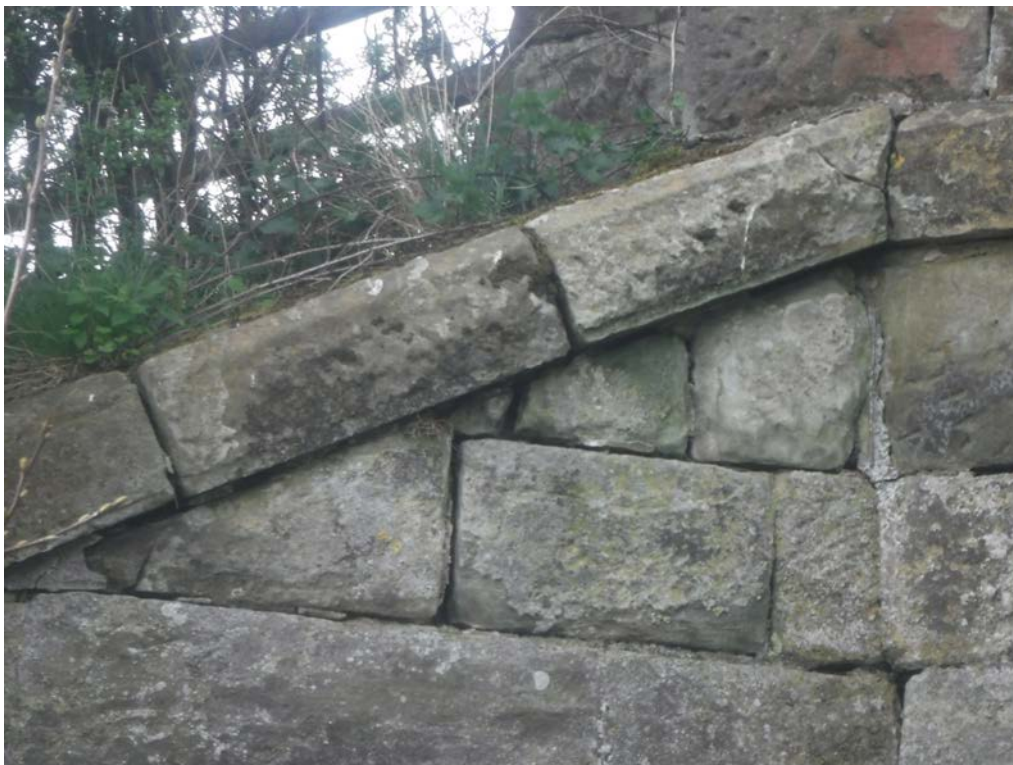
Photo No.16. South East elevation wing wall open joints
