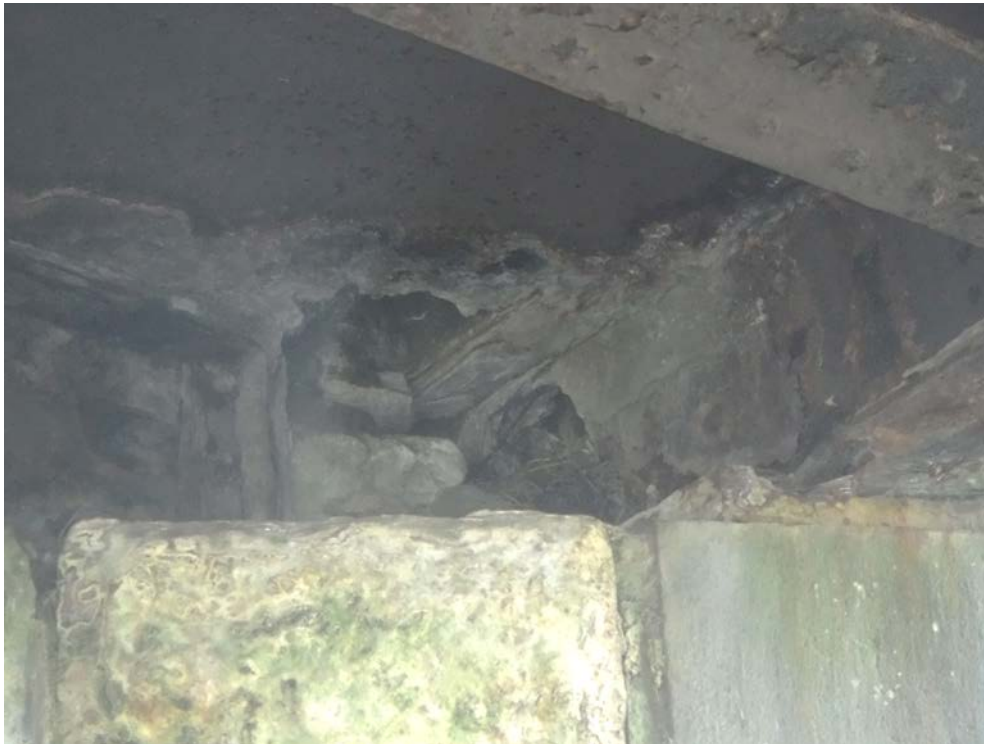
Photo No.15. Deck plate holed
